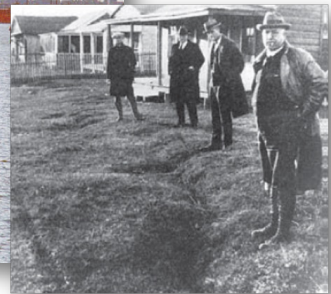
Earth fissures at Goose Creek Oil Field
